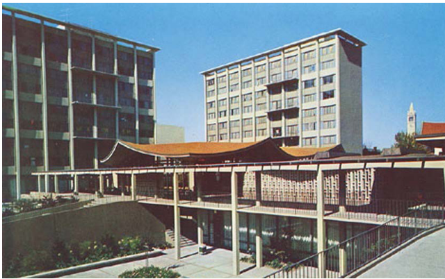
Figure 2. Warnecke and Warnecke, Student Residence Halls, UC Berkeley, 1956 (image in public domain).
